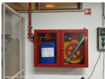
Fire hose reel_Candles.jpg
